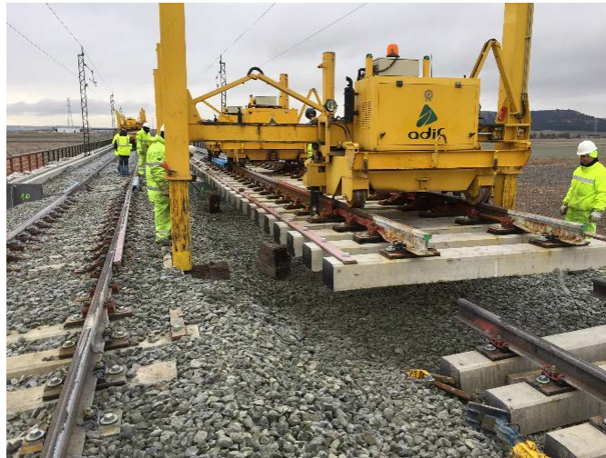
Plate 4.2 Rail panel handling machine
